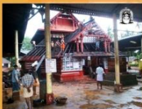
the Garbha Gudi during the renovation
