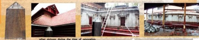
other pictures during the time of renovation
