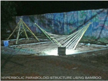
HYPERBOLIC PARABOLOID STRUCTURE USING BAMBOO
